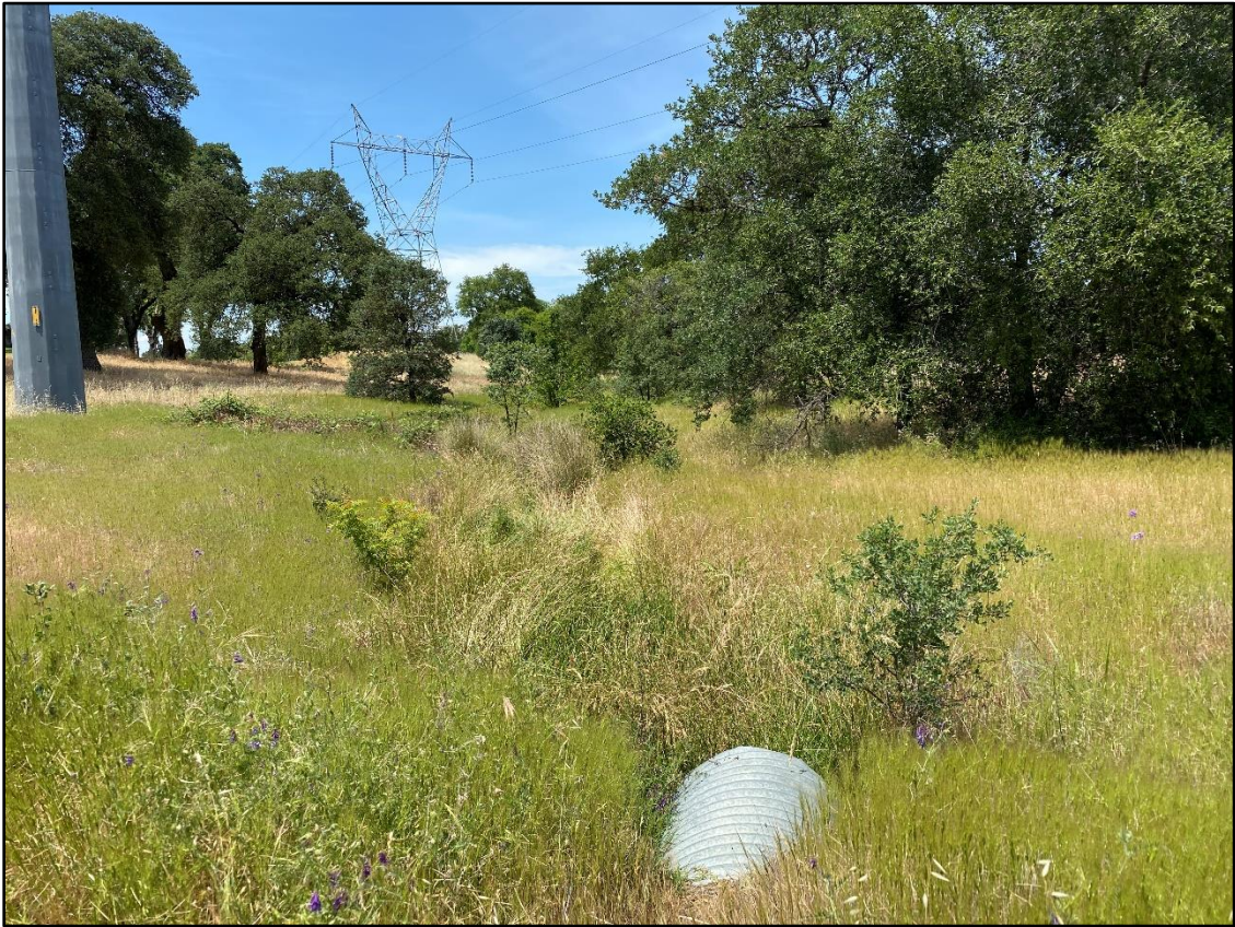
Drainage ditch (DD-1) facing northwest, 18 May 2020
